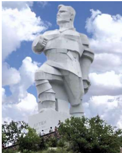
Picture 2. Ivan Kavaleridze. Monument to Artem. 1927. Reinforced concrete. Slavyanogirsk.
